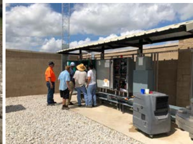
Lift Station controls
