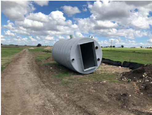
Wet Well at Lift Station under construction
