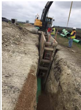
Trenching of line & pipe installation
