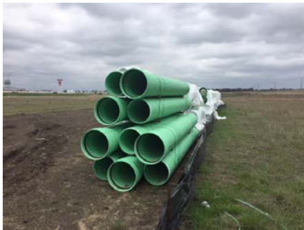
Sewer line pipe
