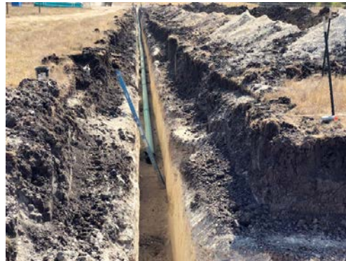
Phase II force main under construction
