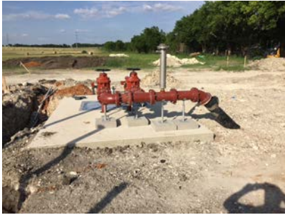
Pump piping within lift station
