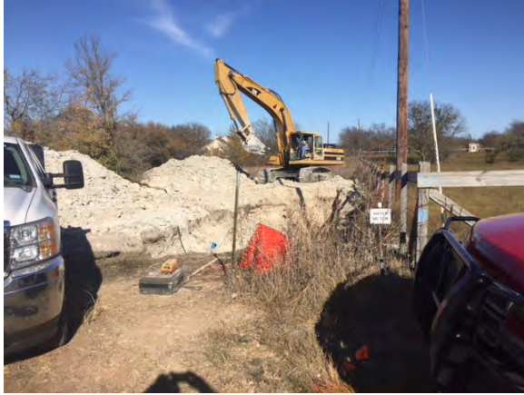
Sanitary Sewer Line Excavation
