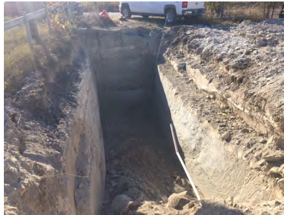
Sanitary Sewer Line Trench
